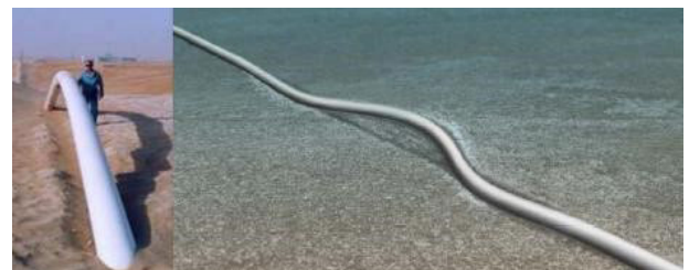
FIGURE 1. Examples of vertical and lateral bucklings of subsea pipelines [4].
